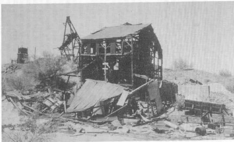
3. The Vulture Mine, Wickenburg, closed over 40 years ago; this structure formed a major exhibit at the Mining Museum in 1982.
