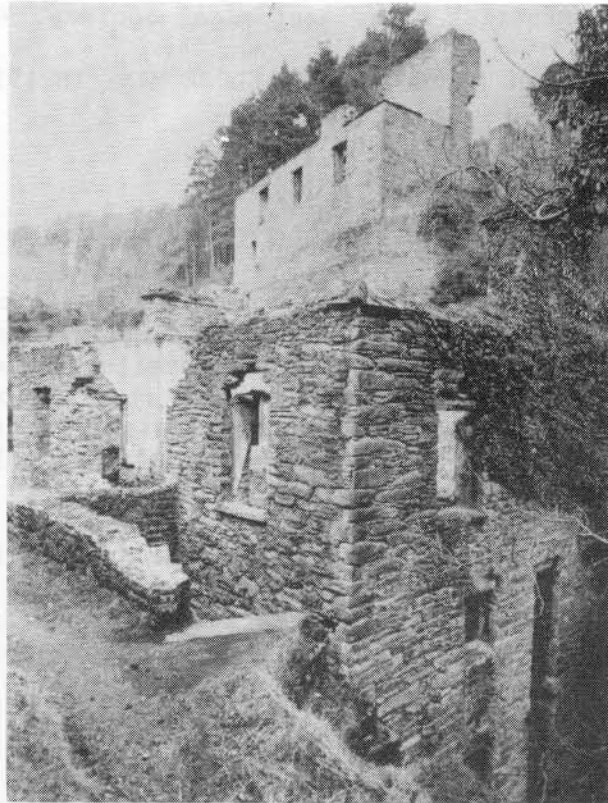
Plate 1 The winding houses at Great Laxey mine. Taken by Anders Jespersen in 1965, looking up the valley. The beam engine house is above. The turbine house is below, and nearer the observer.
