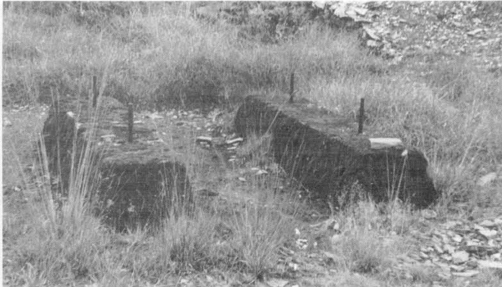
Plate 1. The machine bed for the buddling apparatus, Bell Hole Mine.
