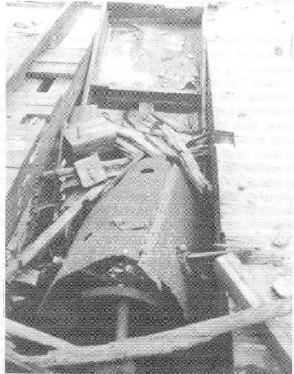
Plate 4 (above). Nantiago, Wales: The wrecked sizing trommel with wooden settling tanks.
