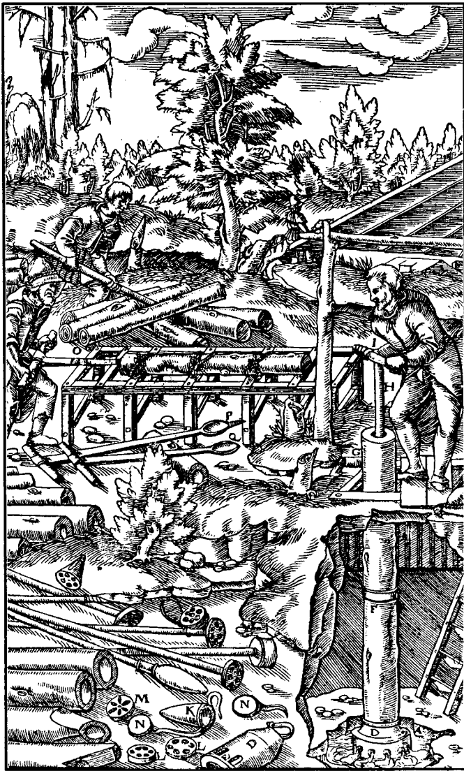
Fig. 4. Boring Pump Trees - Agricola (1556) De Re Metallica .
