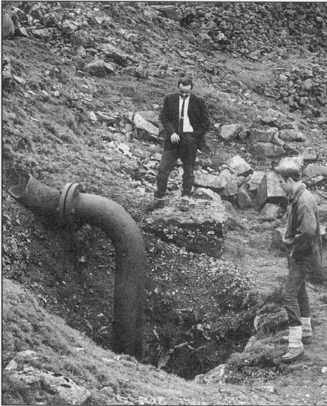
(Above) Remains of the intake pipe which supplied water to the two hydraulic engines 250 feet below.
