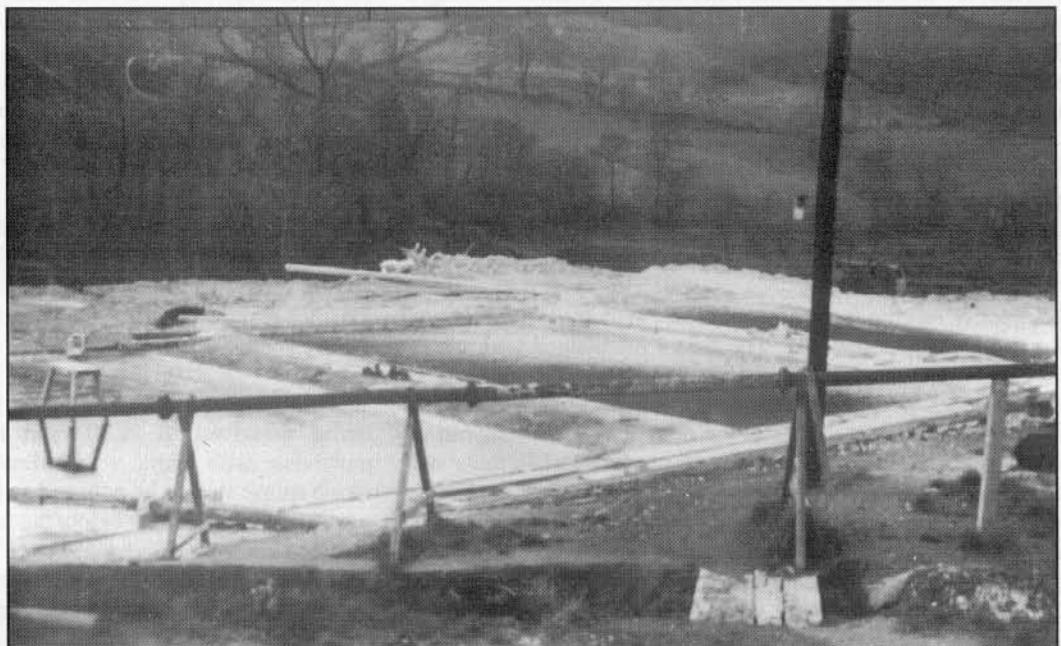
Settling ponds for the calcium sulphate slurry which was then pumped to a waste heap.
