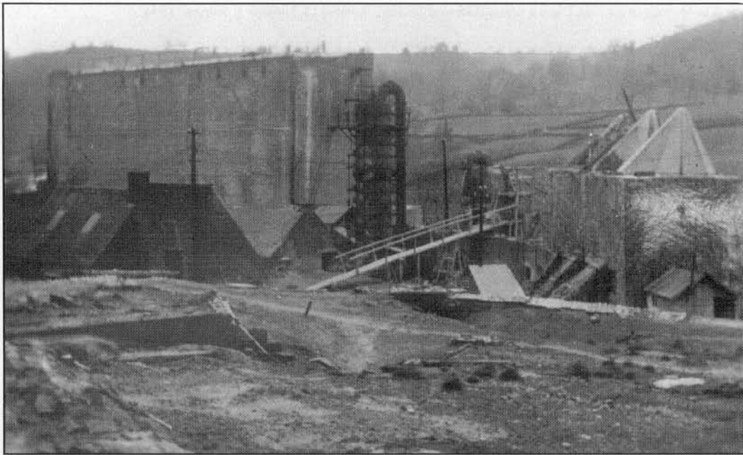
The large condenser (left) 90 by 30 feet by 50 feet high. Gases pass from the tower to three cyclones and then to four scrubbing towers - three together and a fourth just visible between the three and the steel tower. The steel tower was disused.
