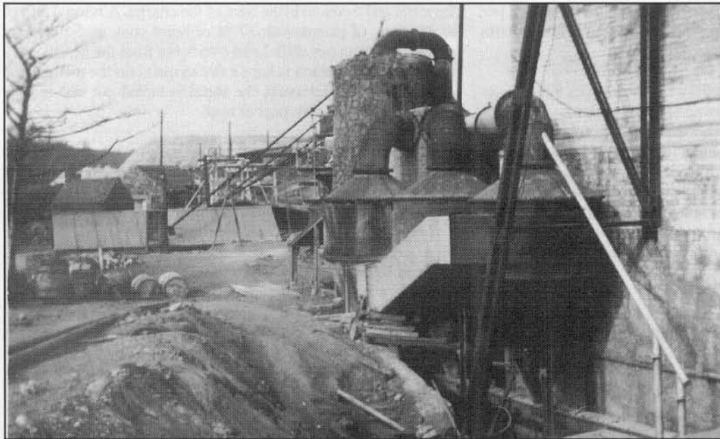
A blower for pumping flue gases at the side of the large condenser.
