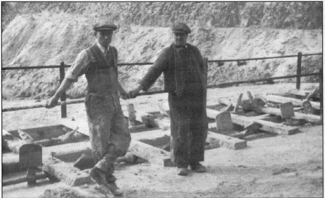
The mixing tanks where the acid-water and lime-water reacted to produce calcium sulphate.
