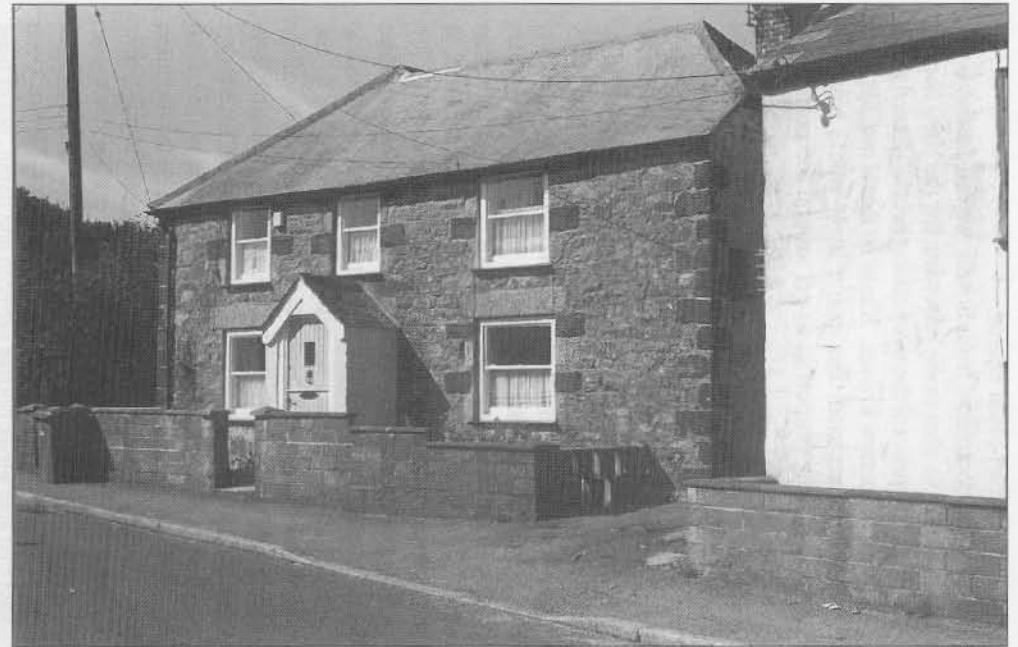
Plate 4. Cottage at Churchtown Rd, Phillack, illustrating the use of slag blocks in the quoins of a building.
