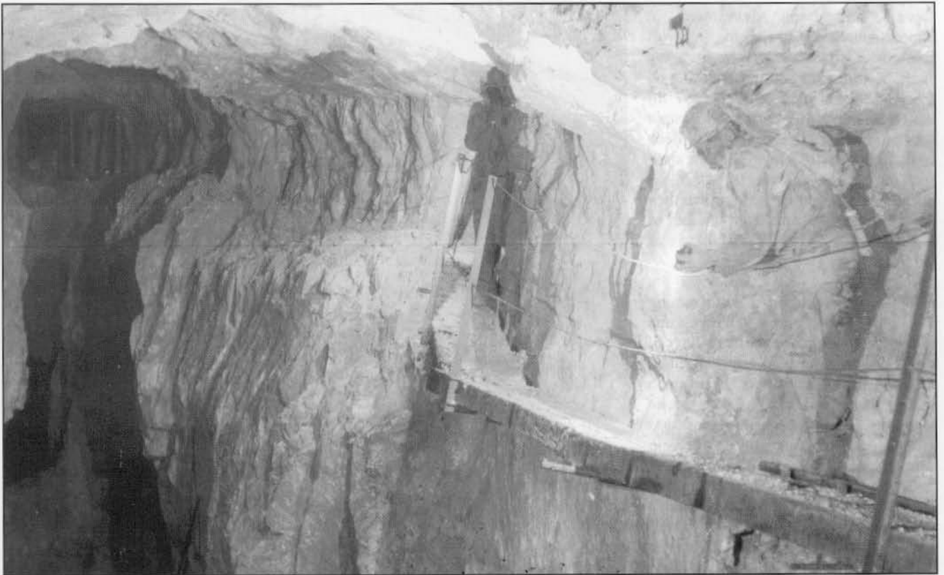
Plate 4. Railway sleepers and rock-cut ledge "catwalk" at the western end of the No. 2 level.
