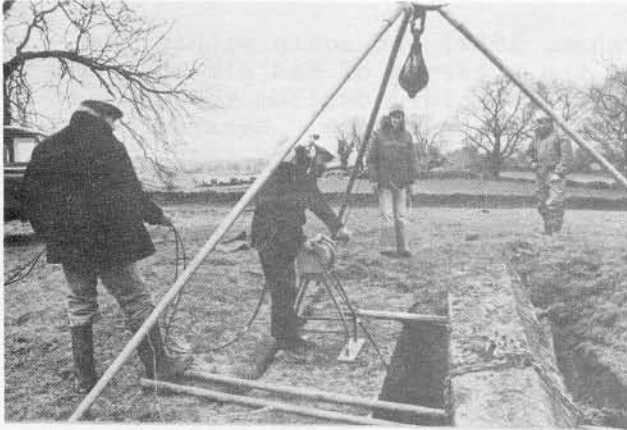
Lowering the lights and camera.
