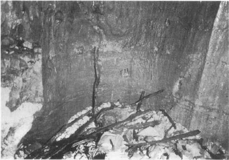
1. Bottom of Round Pitch with fallen stemples on miners' debris and washings with stemple sockets in wall behind.
